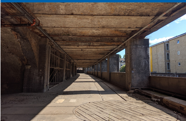
Fig. 3: View down deck level of viaduct.
