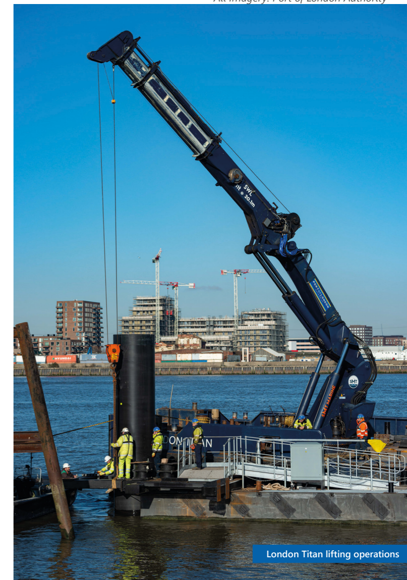
Installation of pile keeps
