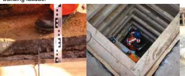
Temporary timber shoring was designed and detailed to support not only the retained ground but also the imposed load from the taxi rank departure road along Eastbourne Terrace. Due to the close passing proximity, other factors had to be taken into account, including access for emergency service and shop delivery vehicles.
